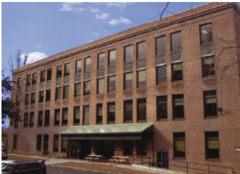
St. Francis Information Technology and Finance Center, 103 Woodland Street - Hartford, CT
